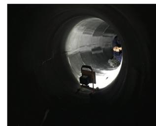
Fig. 5: The finished carbon fibre pipe before nanoceramic coating
