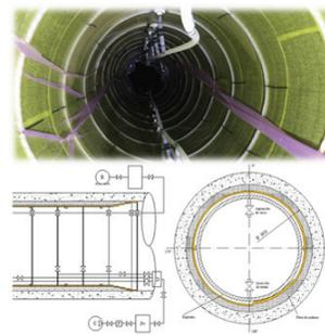
Fig. 4: Infusion and vacuum system, design and installation
