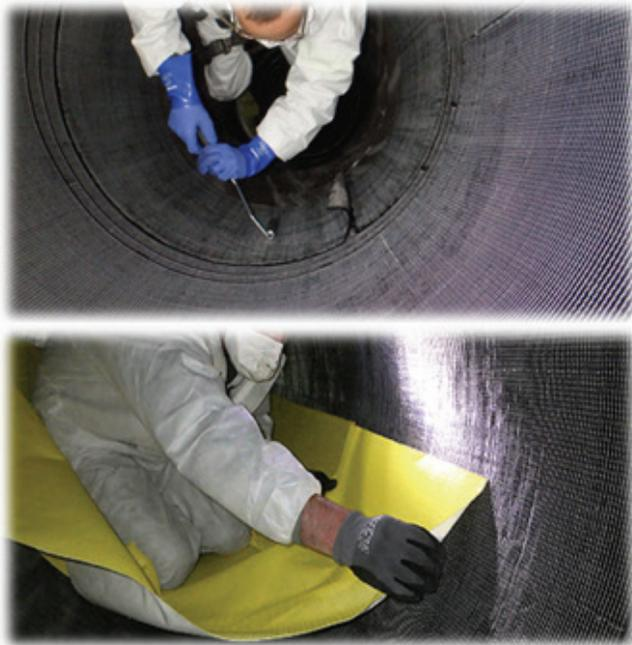
Fig. 2: Installation of the SAERfix carbon non-crimp fabrics (self-adhesive)
